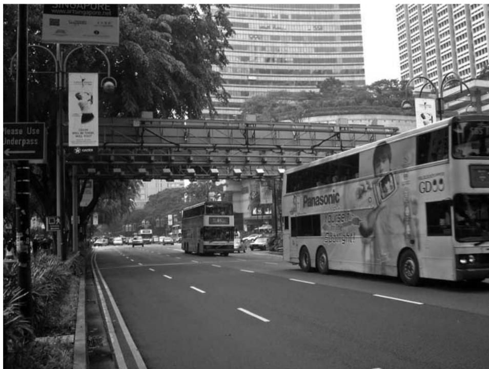
**Figure 7.** Buses pass under an ERP gantry. Cameras for violator detection are visible.
